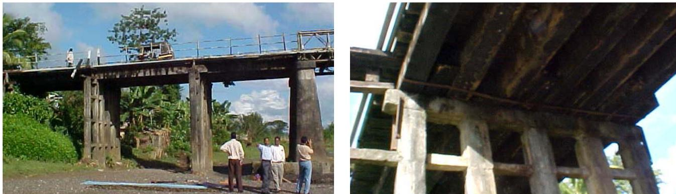
*Figure 35: Kalpong bridge north of Diglipur town has no earthquake resistant features. This deficiency is further accentuated by its poor maintenance.*
