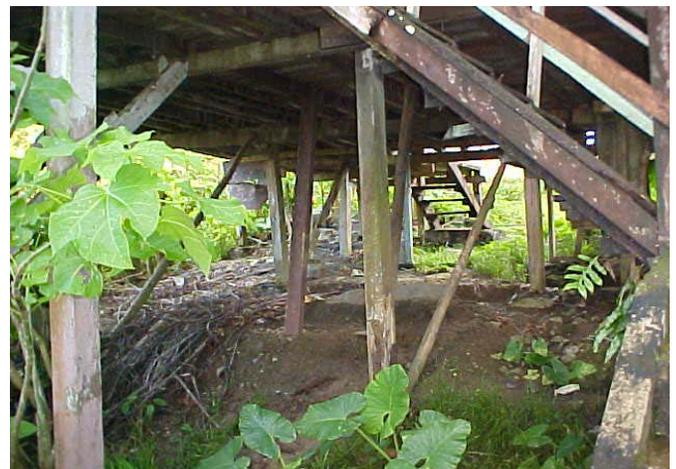
*Figure 13: An old and poorly maintained wooden frame building on stilts on slope with a long history of soil movement and settlement rendered unsafe for further occupation in Diglipur.*
