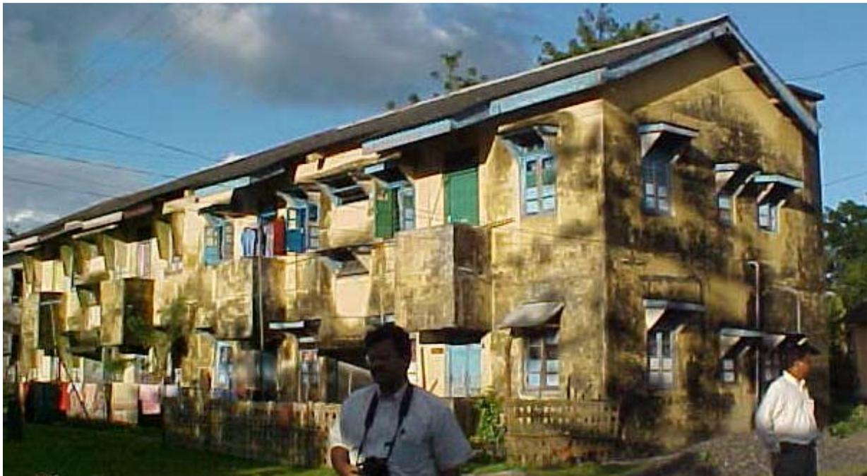
**Figure 23:** Two storey load bearing masonry building for Govt. employees in Diglipur performed satisfactorily despite poor maintenance and upkeep, primarily due to better structural layout and relatively light roof.
