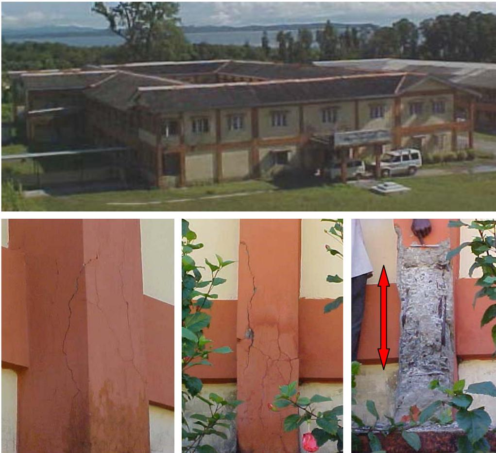
**Figure 18:** Cracking in critical beam-column joint regions due to 'missing' ties for entire beam depth (more than 450 mm) in the main building of Mahatma Gandhi College in Mayabunder.
