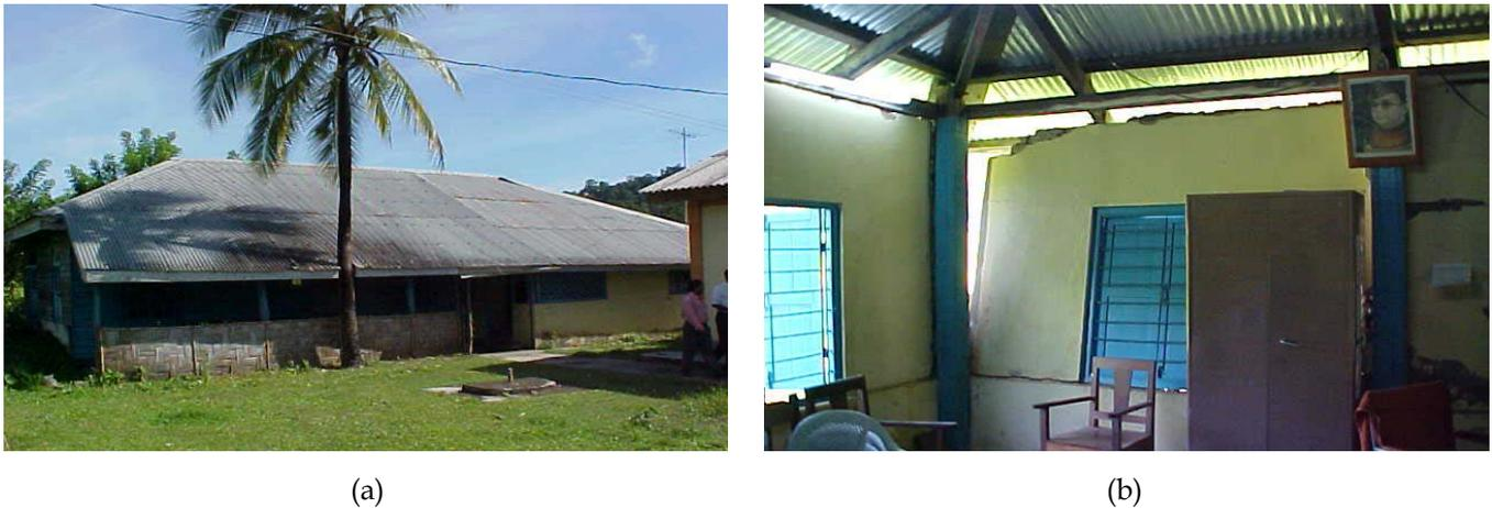
*Figure 14: Masonry bearing wall dislodged out-of-plane due to large movements of flexible roof structure.*
