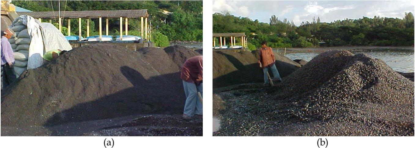
**Figure 10:** Fine and Coarse Aggregates obtained from crushing the sedimentary and basalt rocks available in the region.
