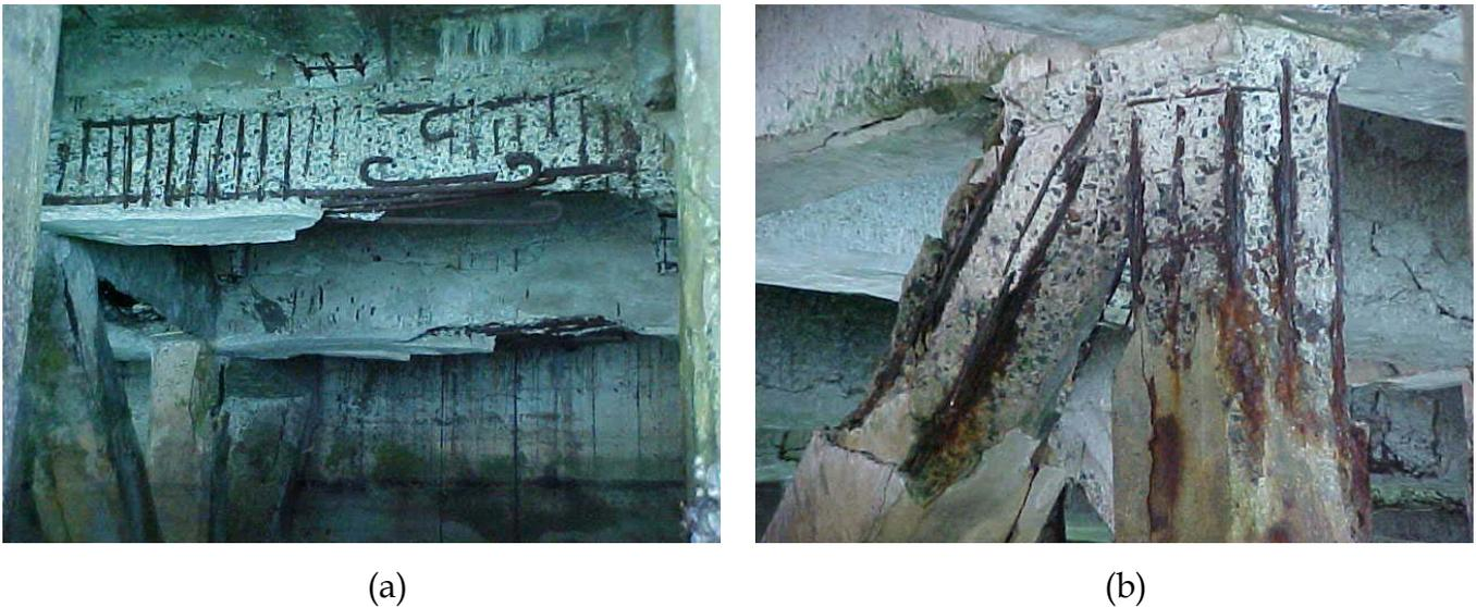
**Figure 27:** Severe corrosion of reinforcing bars and spalling off cover concrete from beams, and (b) columns and batters.
