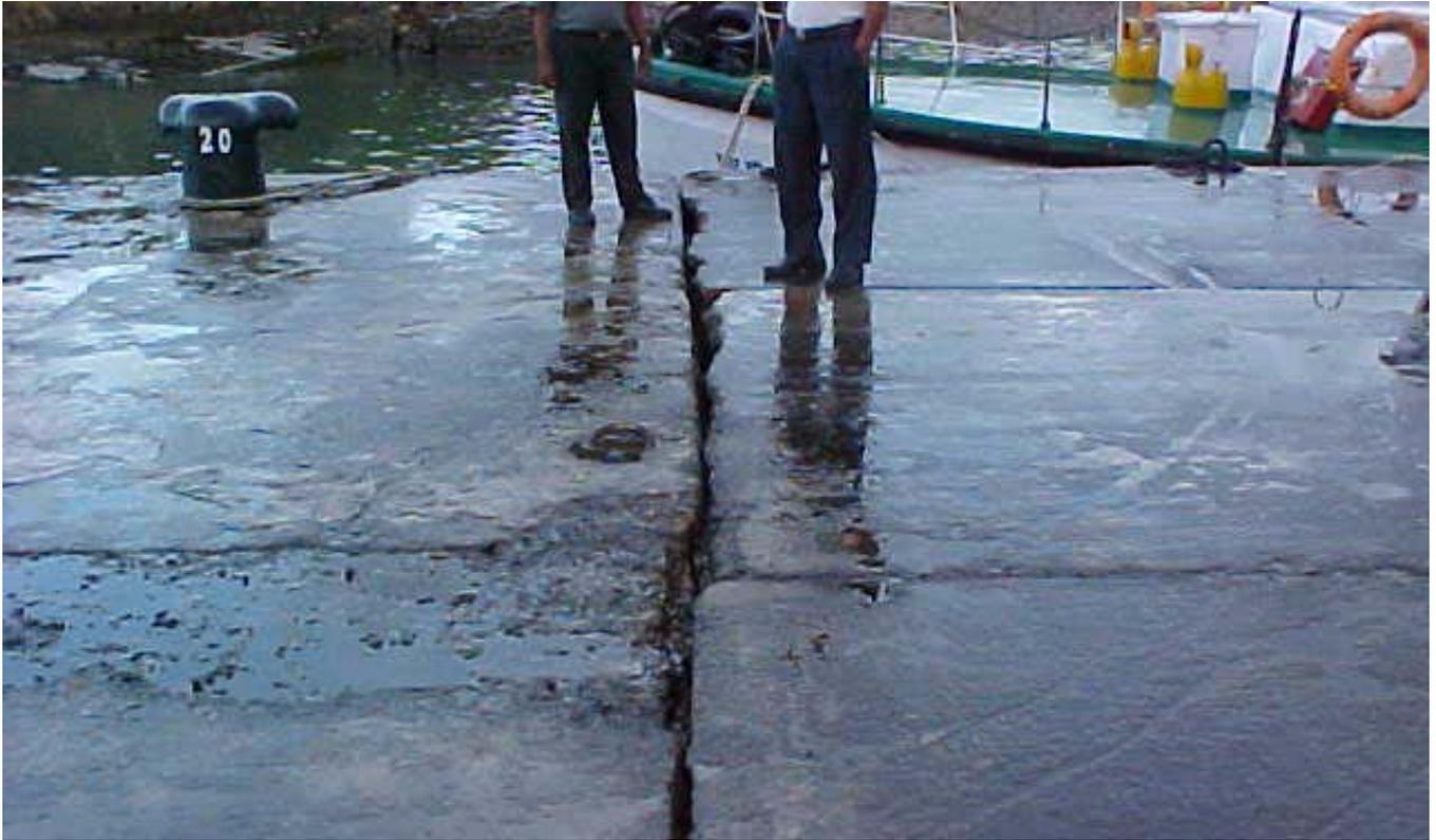
*Figure 31: Pounding damage at the expansion joints on the main jetty.*
