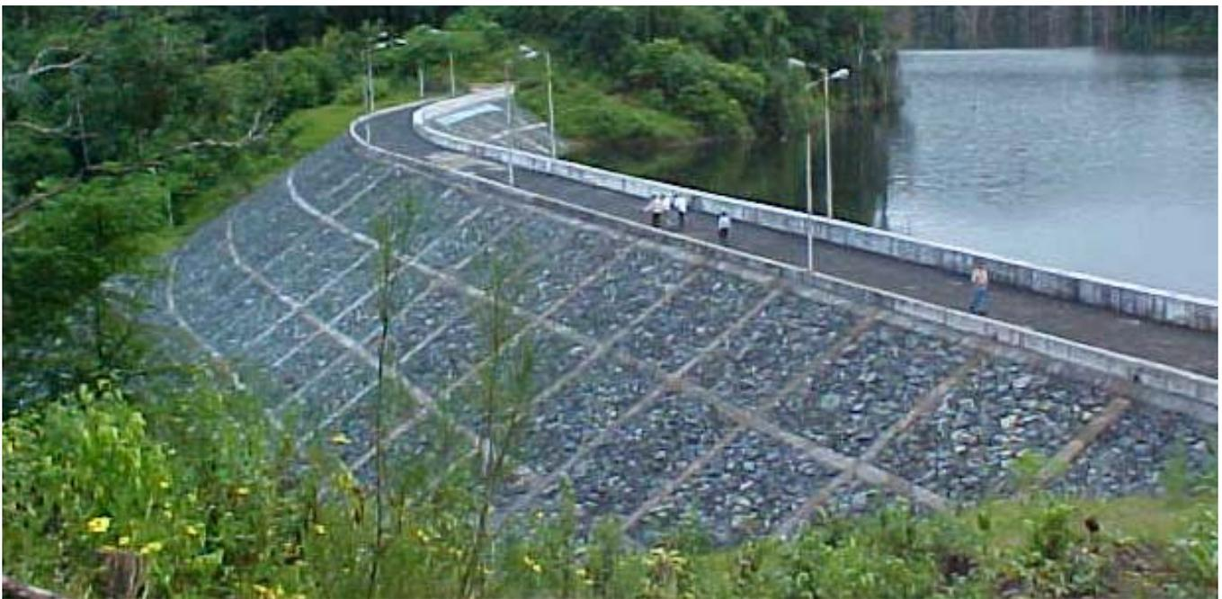
*Figure 33: Concrete and rockfill dam on the left and right fork of the Kalpong river.*
