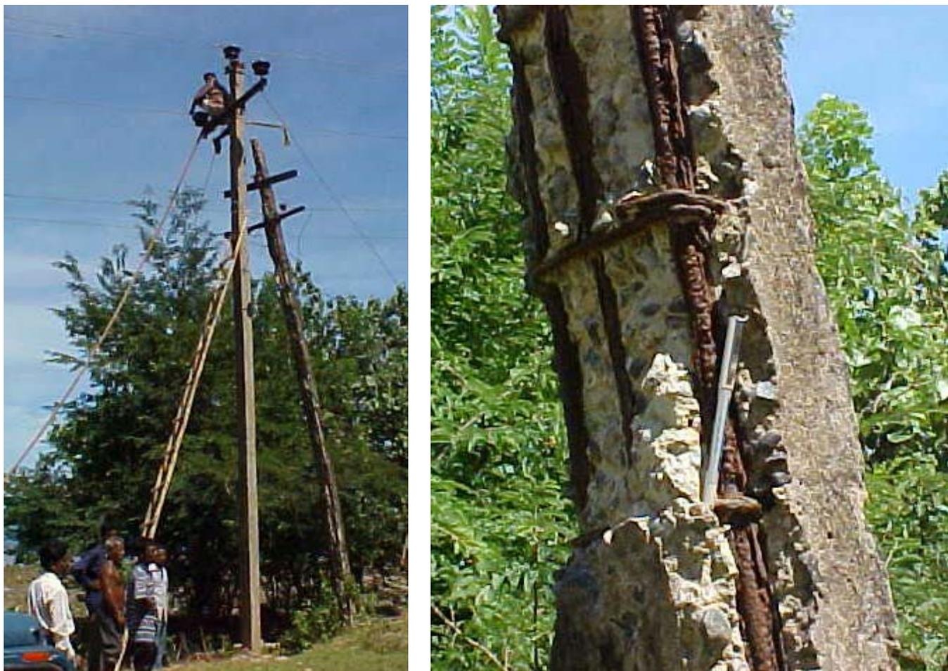
*Figure 37: Deteriorated RCC electric poles gave way in the area of major shaking disrupting power supply.*
