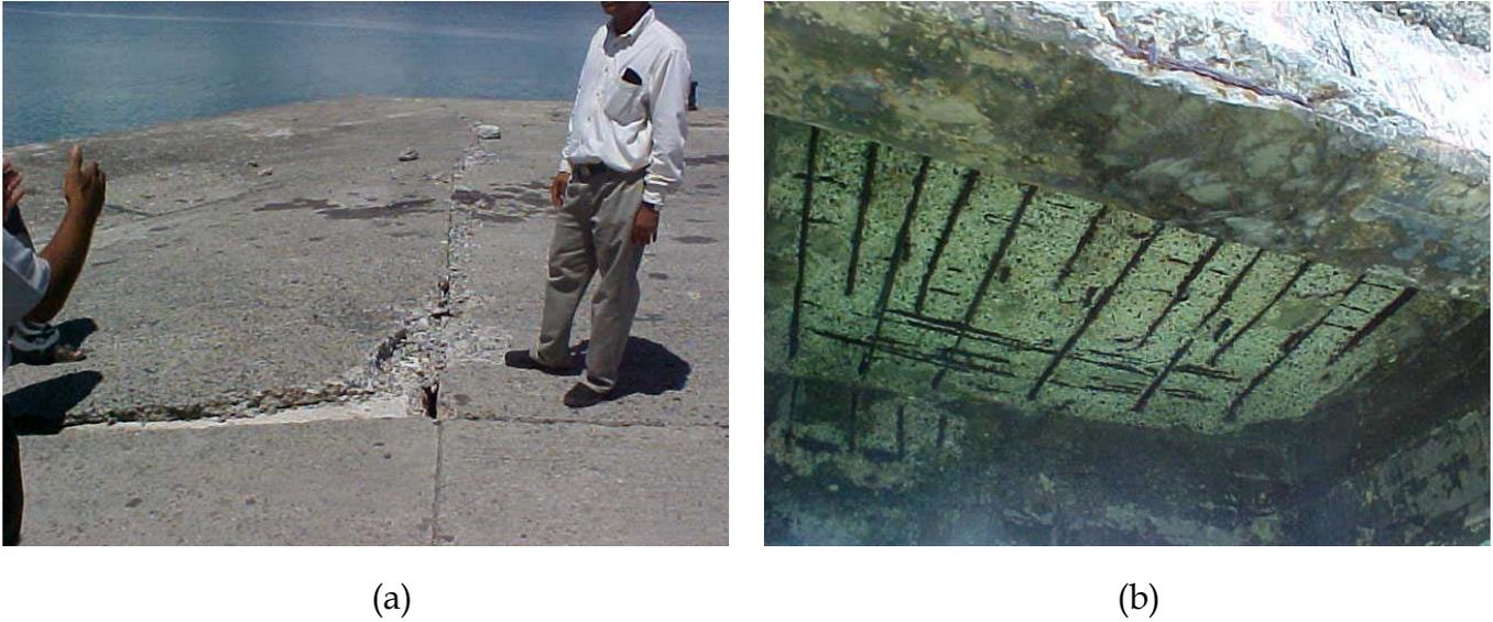
**Figure 26:** (a) Pounding damage at the intersection of approach to main jetty at the top, and (b) exposed slab reinforcement underneath due to heavy corrosion.
