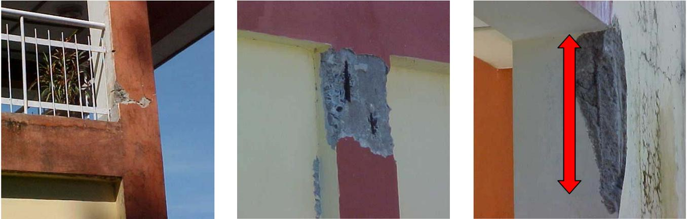
**Figure 20:** Damage to columns, which reveal absence of transverse ties over a length of about 450 mm from the beam soffit. This omission during the construction compounded with poor architectural planning and configuration resulted in significant damage in an area that sustained less than moderate shaking.
