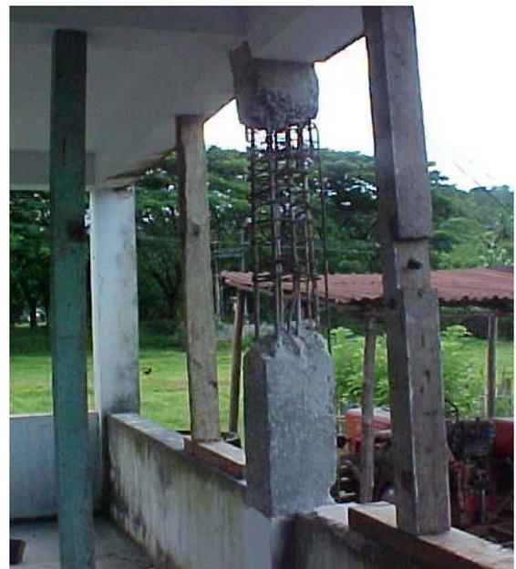
*Figure 38: Inadequate repair of damaged columns of the Panchayat building at Nabagram village.*
