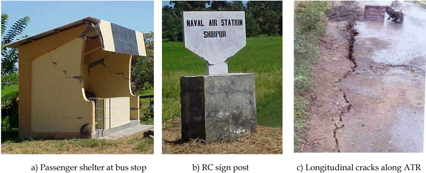
**Figure 5:** Damage due to significant shaking in Shibpur area near shoreline in Diglipur.
