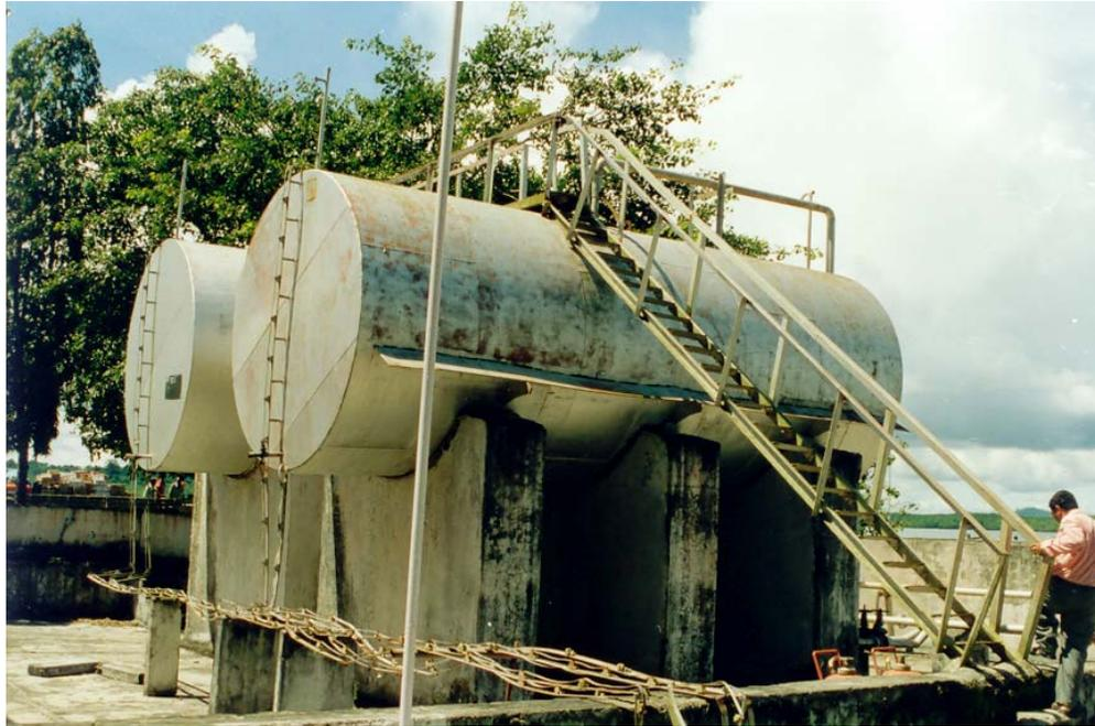
*Figure 28: Cylindrical tanks for Petrol, Lubricants and Oil (POL) at Diglipur harbour.*
