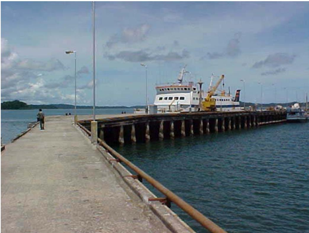
*Figure 24: Approach jetty meeting an angle with the main berthing jetty at Diglipur harbour. The damage to jetty slab was concentrated at the intersection.*
