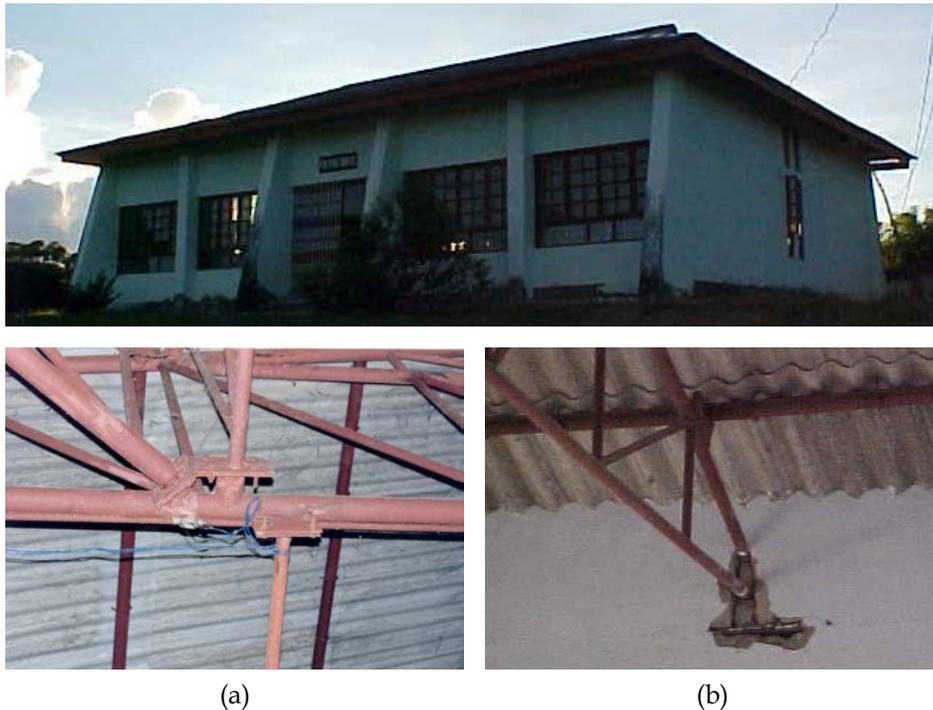
*Figure 15: Poorly detailed joints between truss pipe members, and between the truss and the supporting RC column.*
