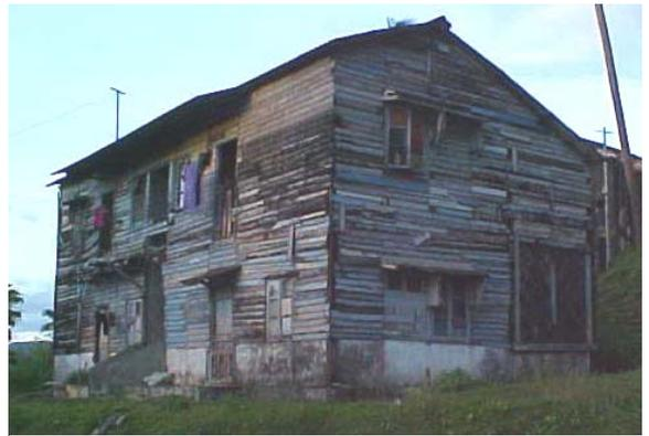
*Figure 12: An old 2-storey timber house in dilapidated condition; numerous such constructions stand vulnerable under expected strong shaking in the region.*
