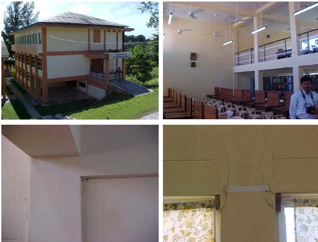
**Figure 21:** Cracking in the joint region of columns in the asymmetric library building at Mahatma Gandhi College in Mayabunder.
