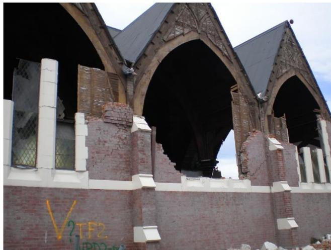
*Figure 4. An earthquake has destroyed most of the brick cladding and glazing of this building.*
