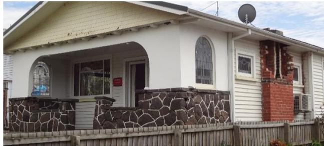
*Figure 3. A brick chimney has broken off at roof level and fallen. Most of the remaining chimney is damaged (N. Allaf).*
