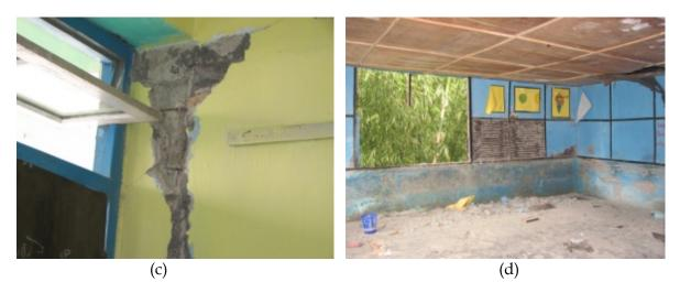
**Fig. 14.** Damage observed at Government Secondary School at Sichey (a) old school building, (b) additional school building, (c) damage to RC columns, and (d) damage to Ikra walls on top floor (Photo: Hemant Kaushik)
