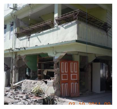
**Fig. 12.** Complete damage of columns and exterior wall in a building at Chungthang due to poor detailing of column reinforcement, lack of confining reinforcement, improper splicing of rebars, inferior detailing of columns with corbel (Photo: Tripti Pradhan)
