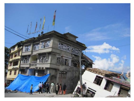
**Fig. 7.** Collapse of two multistory RC frame buildings at Balwakhani, Gangtok (Photo: Tripti Pradhan)
