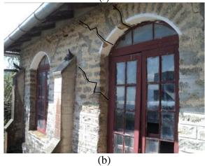
**Fig. 13.** (a) Damage reported at Kalimpong Girl's High School (b) Damage to semi-circular arches, diagonal cracks in masonry pier (Photo: Keya Mitra)
