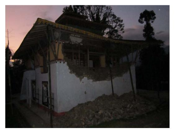
**Fig. 18.** Partial collapse of stone masonry walls of a Monastery temple at Mangan (Photo: Goutam Mondal)
