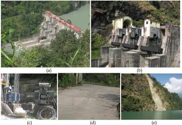
**Fig. 20.** Concrete gravity dams in operation at (a) Project Teesta-V, and (b) Project Rangit, (c) damaged electrical transformer at Teesta-V dam site, (d) ground deformation at Teesta-V dam site, and (e) accumulation of excessive debris and silt in reservoirs due to landslides (Photo: Kaustubh Dasgupta)
