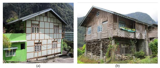
**Fig. 9.** Traditional construction type (a) Ikra house (Photo: Vaibhav Singhal) (b) Shee-Khim house (Photo: Neha Parool)
