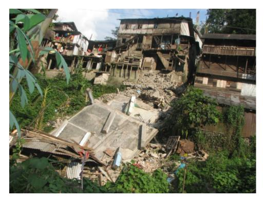
Fig. 8. Collapsed four story reinforced concrete building at Dikchu Bazaar (Photo: Hemant Kaushik)
