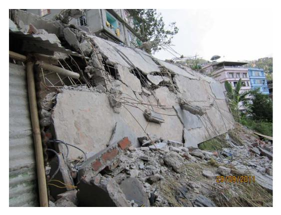
**Fig. 10.** Complete collapse of newly constructed RC building at Lumshey Basty, Gangtok (photo: Neha Parool)
