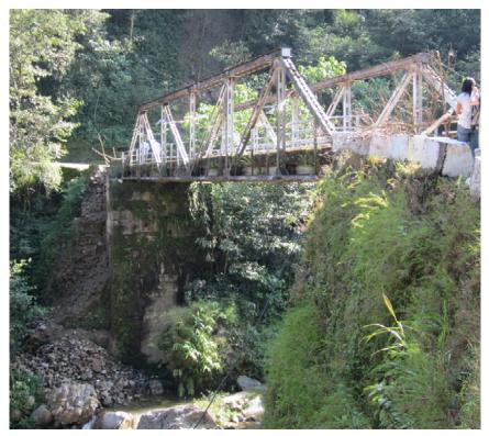
Fig. 15. Damage to the wing wall of steel truss bridge on Raykhola (photo: Tripti Pradhan)
