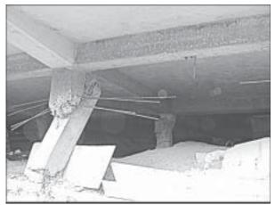
Fig 6 Collapse of three-storey reinforced concrete frame building at Port Blair (Photo: Sudhir K Jain)
