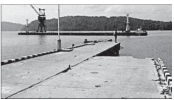
Fig 7 Collapse of the 80-m segment of the approach to Great Nicobar island jetty at Cambell Bay. This has adversely affected the relief work (Photo: CVR Murty)
