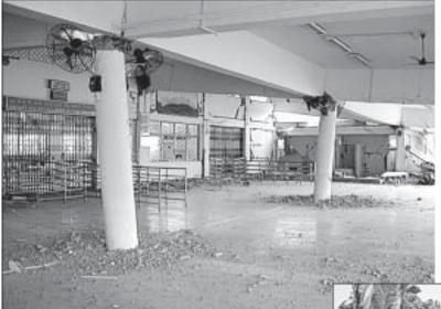
Fig 3 Collapse of a stilt plus one-storey house in reinforced concrete near Port Blair (Photo: Sudhir K. Jain)
