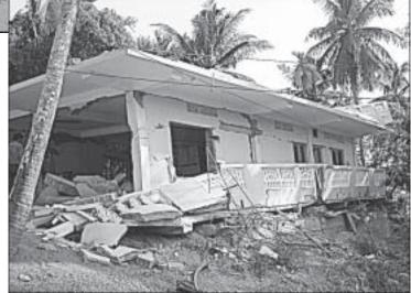
Fig 4 Collapse of a stilt plus one-storey house in reinforced concrete near Port Blair (Photo: Hemant Kaushik)
