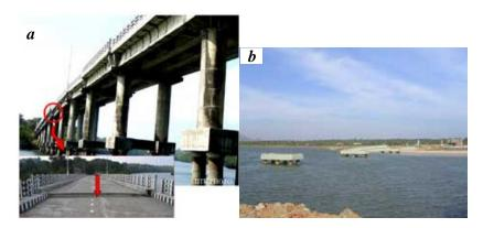
**Figure 6.** *a*, Three middle spans of Chengappa Bridge over Austen Strait connecting Middle Andaman and North Andaman Islands, 230 km north of Port Blair fell off from the bearing due to ground shaking. (Photo: Durgesh C. Rai). *b*, Complete loss of spans of the four-span RC bridge at Melmannakudi due to tsunami. (Photo: Alpa Sheth).
